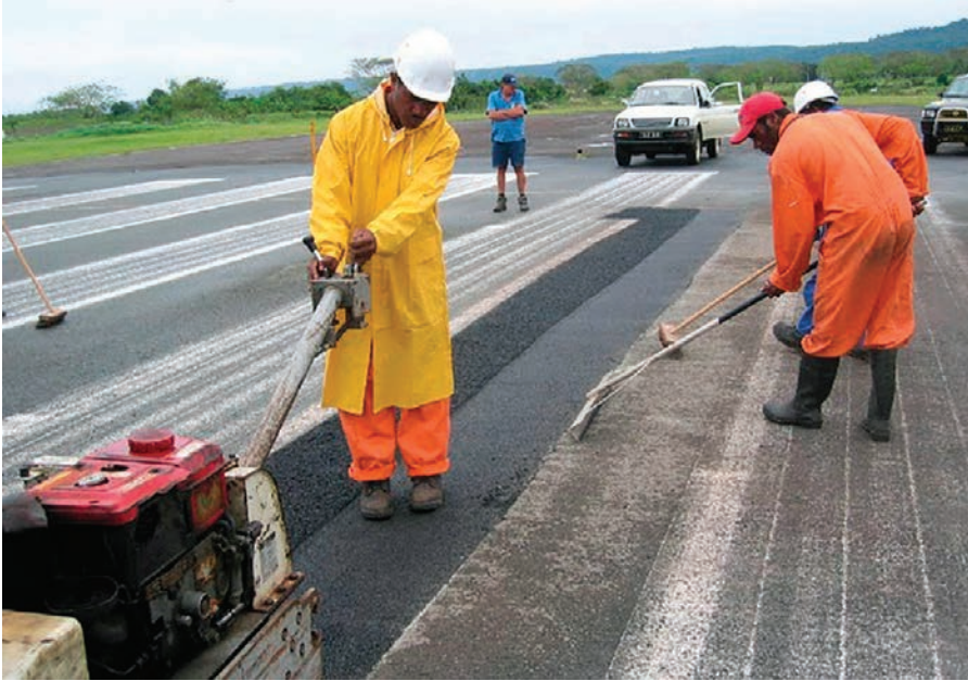
At left, workers apply cold mix asphalt on an airport runway in the South Pacific. Above, cold mix asphalt is used to create a mining road in Chile.
