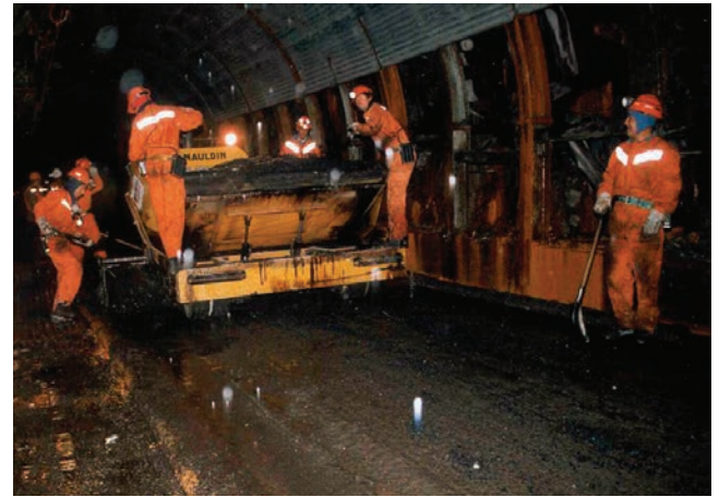
At left, workers apply cold mix asphalt on an airport runway in the South Pacific. Above, cold mix asphalt is used to create a mining road in Chile.
