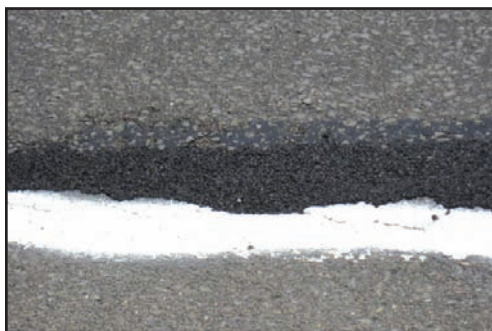
The seam ranged in size from ½ to 4 inches deep and up to 6 inches wide.
