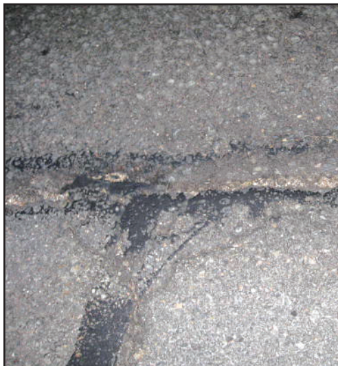
The seam ranged in size from ½ to 4 inches deep and up to 6 inches wide.
